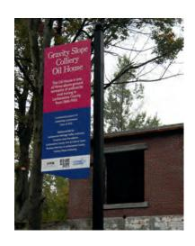
The Restore the Slope project renovated one of three historic buildings on the Gravity Slope Colliery site in Archbald. Known as the "Oil House," LL orchestrated roof repair, ceiling construction, door and window replacement, brickwork, graffiti removal, painting, stairs, exterior site clean-up, and landscaping.
